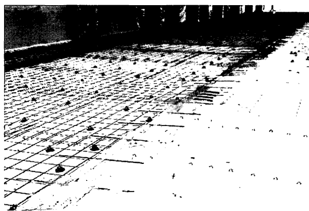
Figure 8.11: Permanent formwork, with dowel bars in place, for a formed restrained-movement joint in a long strip construction. The walls and columns are protected with polythene.
